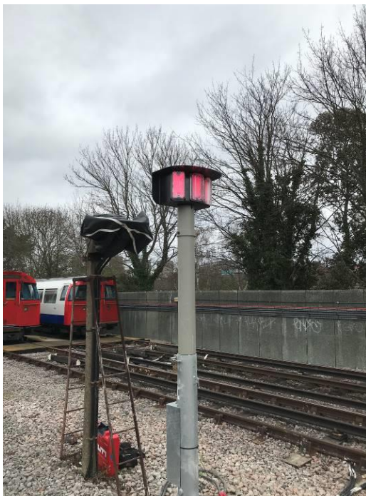
Figure 2: Old (bagged, left) and new stop light / Light illuminated at night
