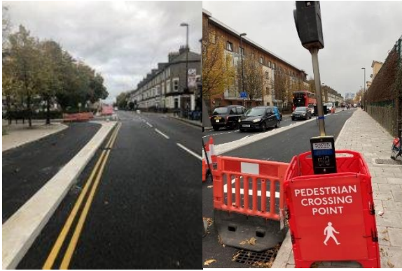
Image 1: C4 Evelyn Street construction
