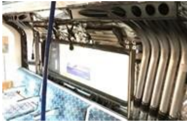
Figure 1: Installation trials of a new pressurised ventilation system
