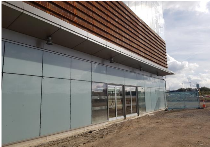
Figure 3: Station Glazing works and platform finishes being installed (above and below)
