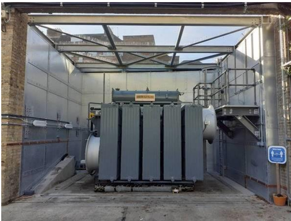
Image 1: New HV Coupling Transformer installation at Stockwell sub-station
