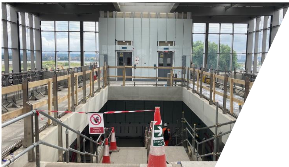
Figure 4: Lift installation complete three months behind schedule
