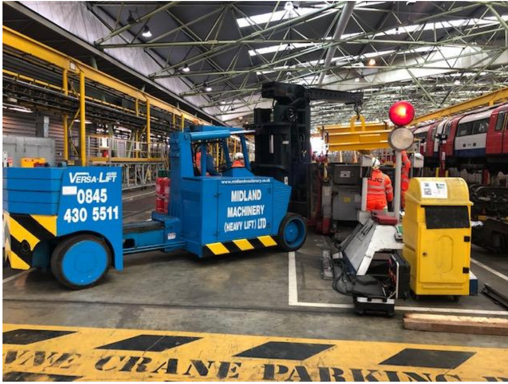
Images 2 and 3 - Mobile wheel lathe installation at Stratford Market depot Jubilee line
