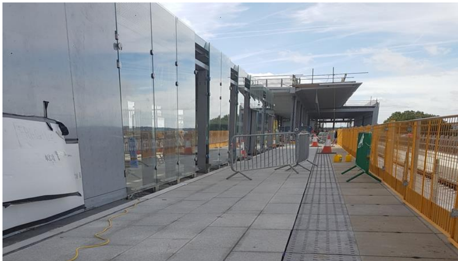
Figure 3: Station Glazing works and platform finishes being installed (above and below)
