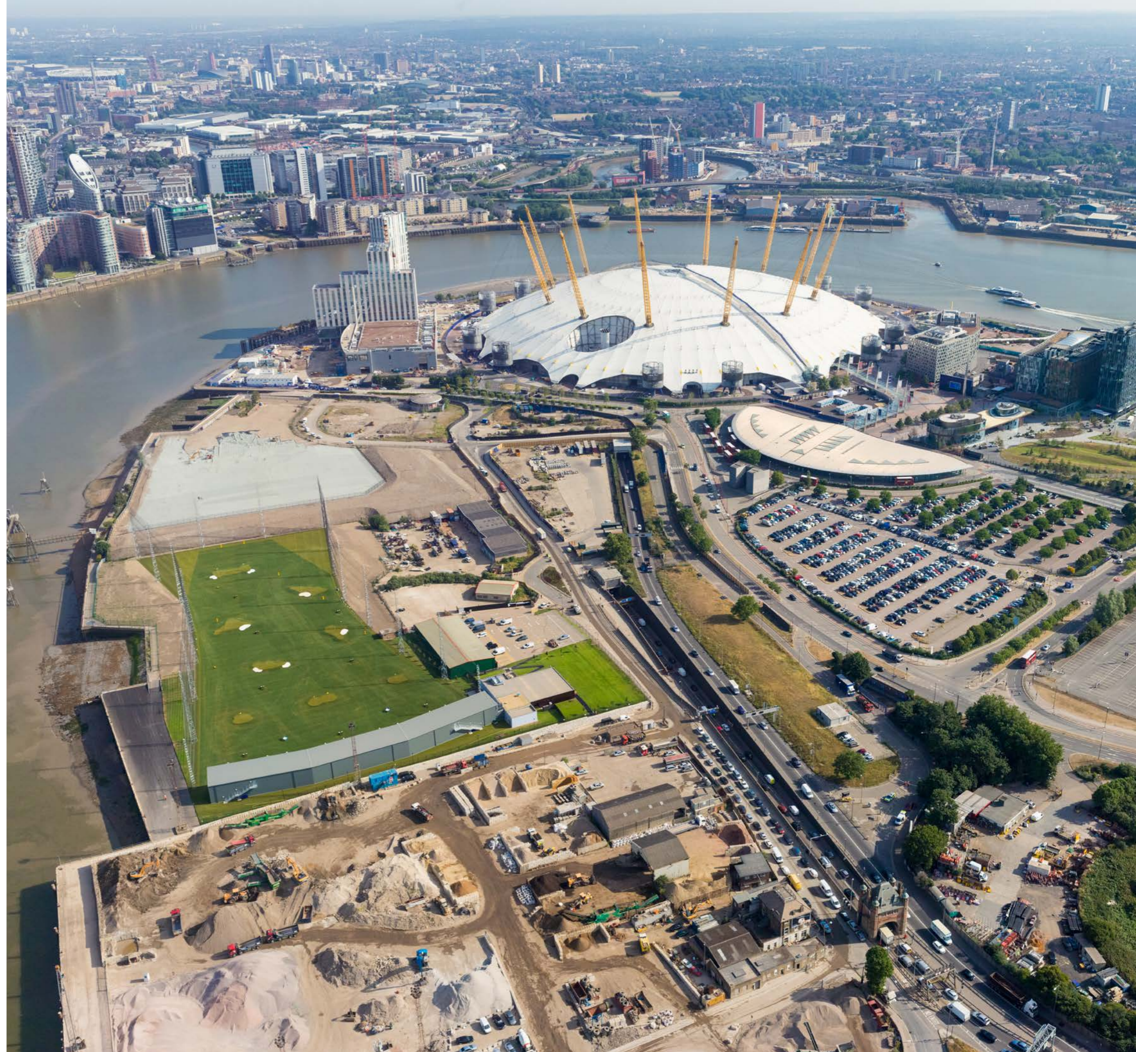
Construction work on the Silvertown Tunnel is progressing well
