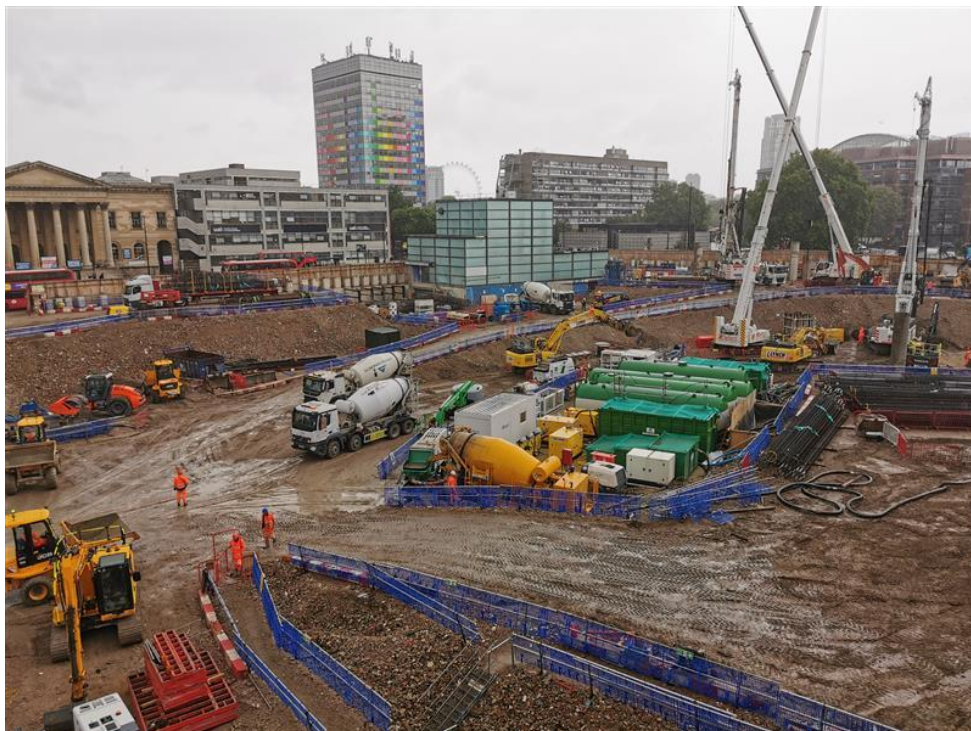
Figure 3: Developer works on the new station box at Elephant & Castle
