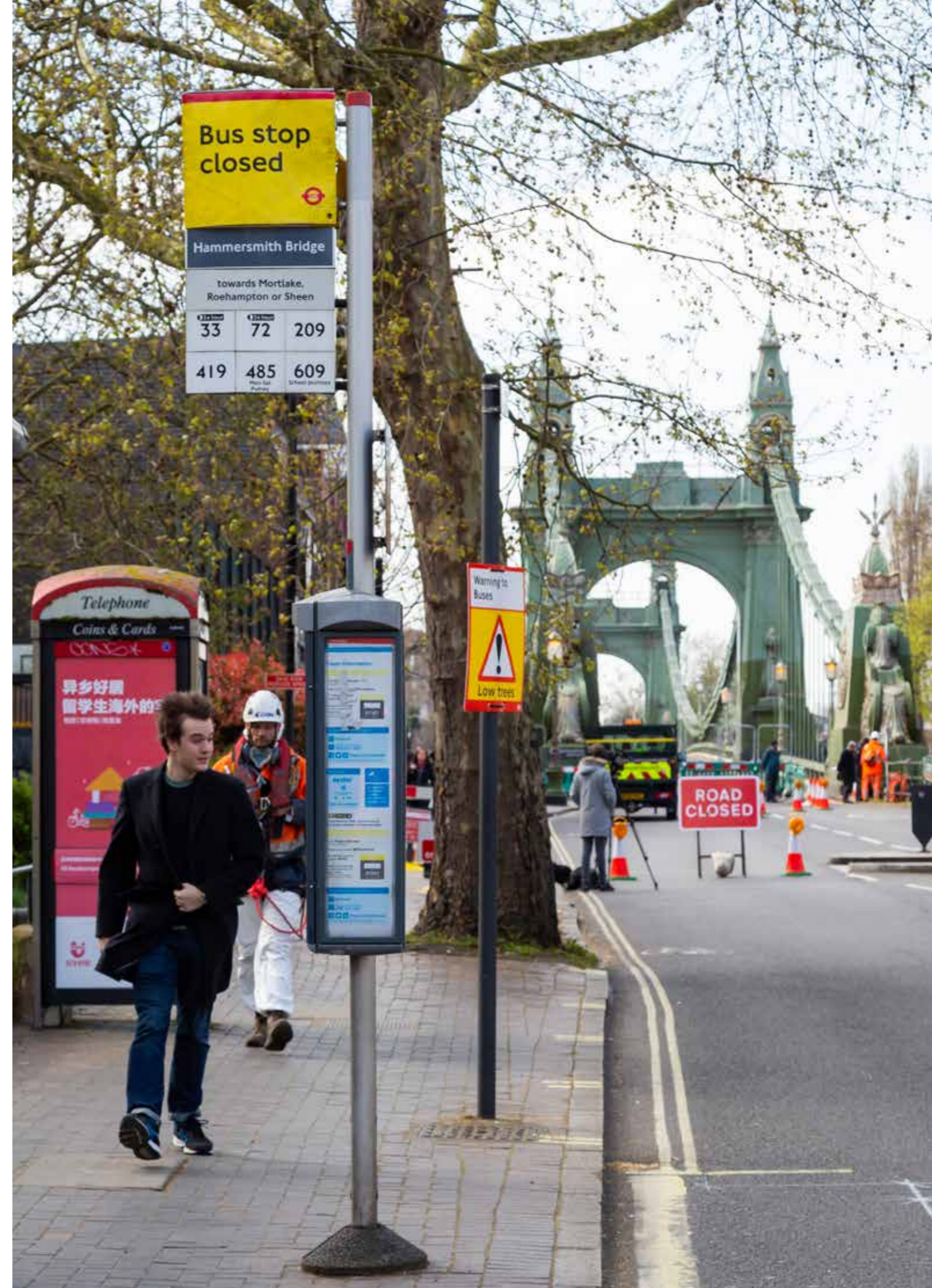
Hammersmith Bridge stabilisation work is under way
