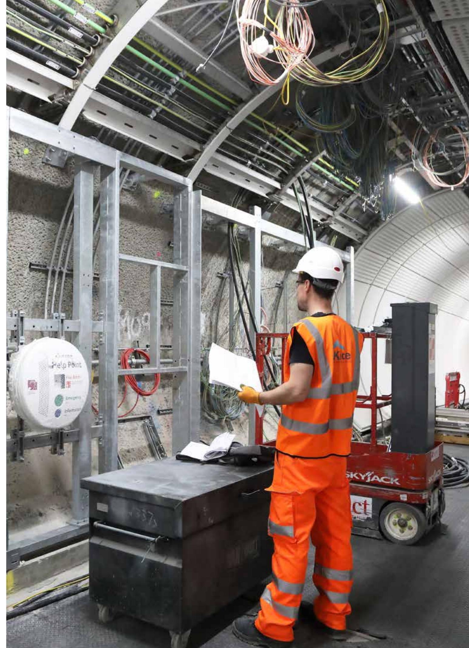
We are continually monitoring and assessing our huge asset base
