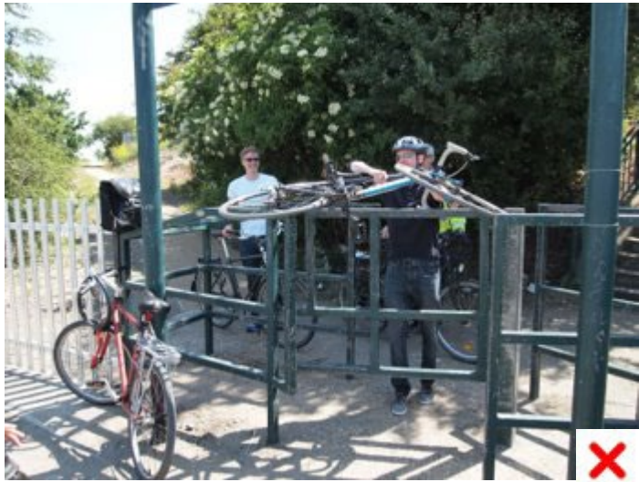
Obstructive railings on cycle path
