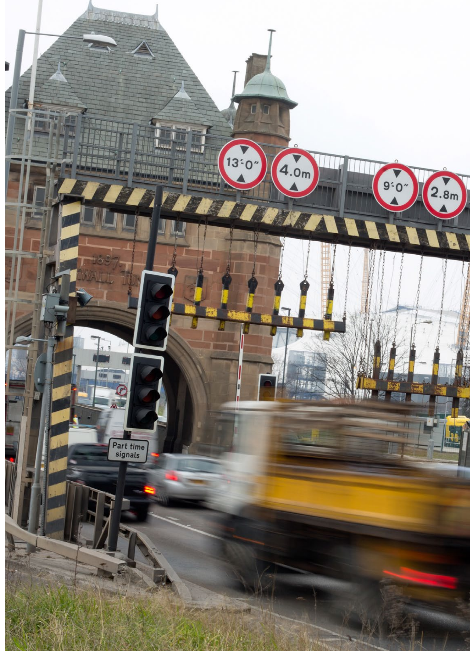
We are renewing critical systems in the Blackwall Tunnel
