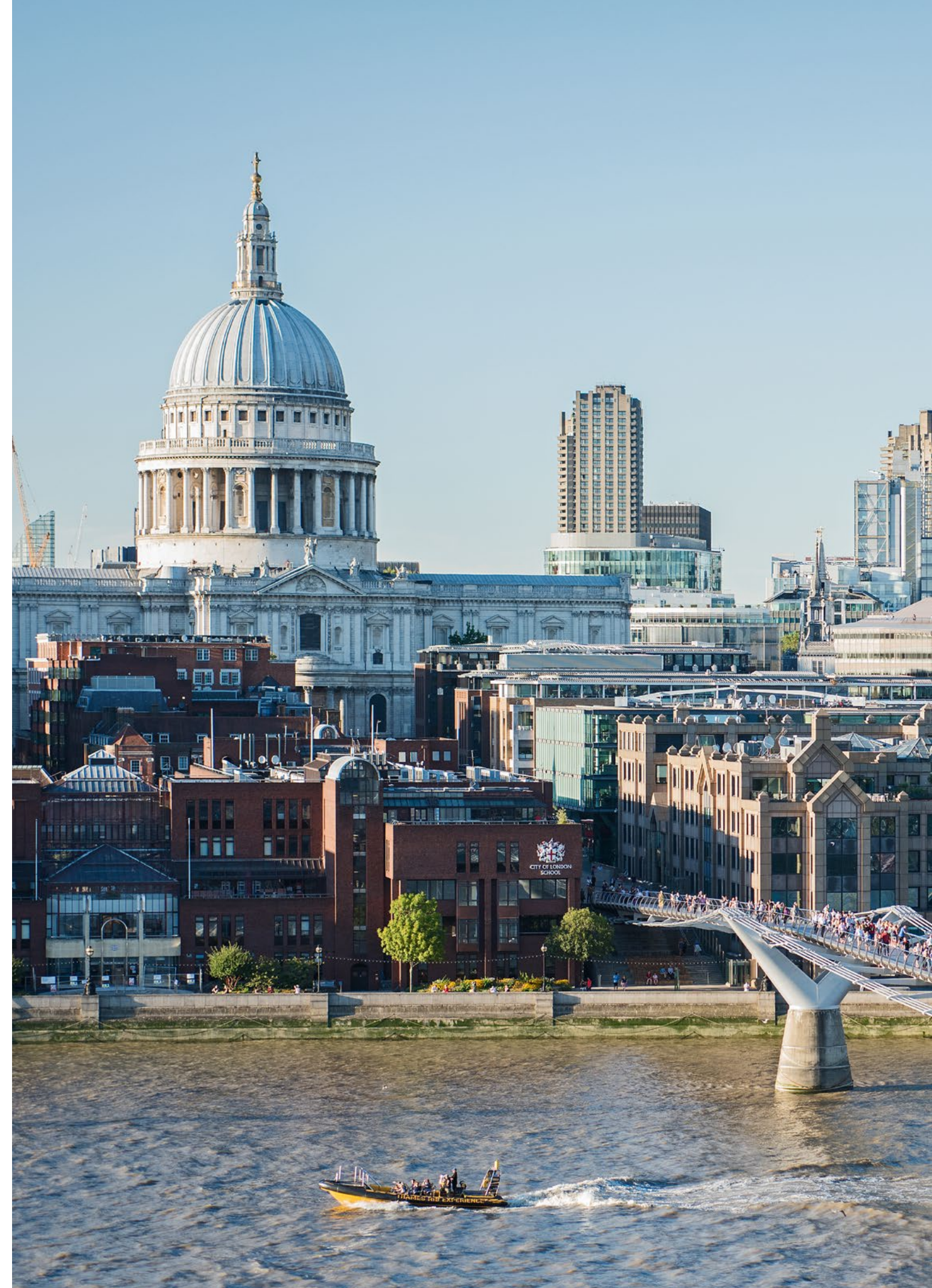
Work is ongoing to address water ingress issues at St Paul's station
