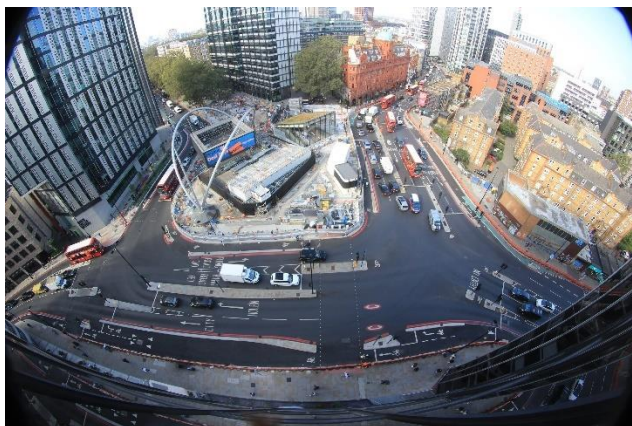
Figure 6 – Old Street highway works substantially complete
