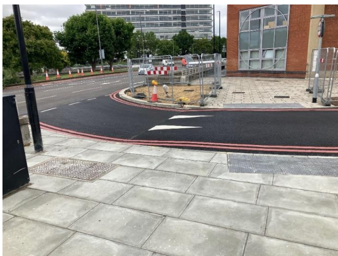
Figure 7 – Tolworth progress: Barnsbury Road raised table
