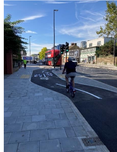
Figure 3 – Cycleway 9 Kew Bridge junction to Waterman's Park
