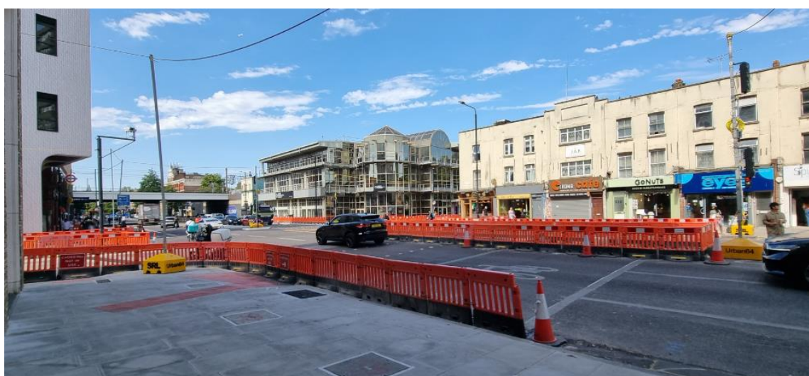
Figure 9 - Construction underway on Holloway Road Safer Junction
