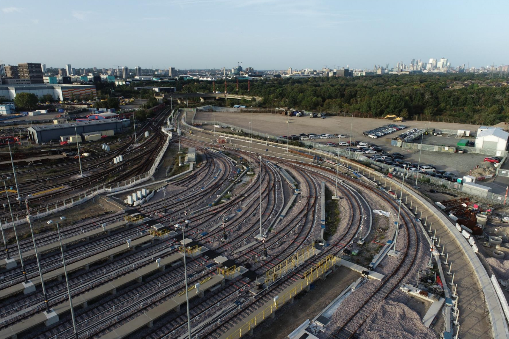
Northern Sidings construction progress – works substantively complete
