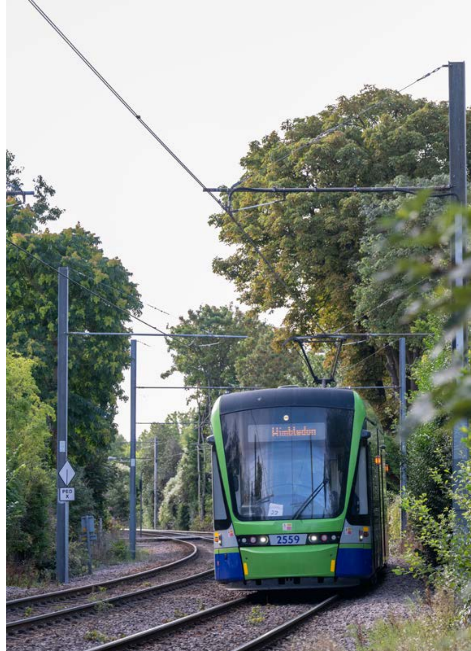
We have upgraded our communications equipment
