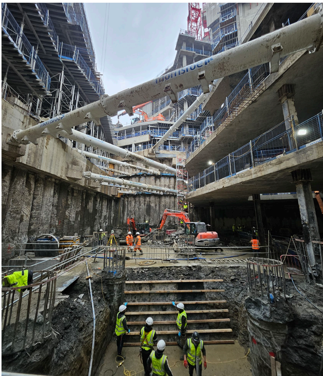
Figure 44: The new station box at Elephant & Castle excavated to its lowest level, 33 metres beneath ground level. Source: TfL
