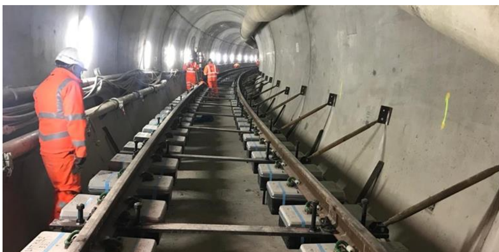
Figure 1: Civils and track progress
