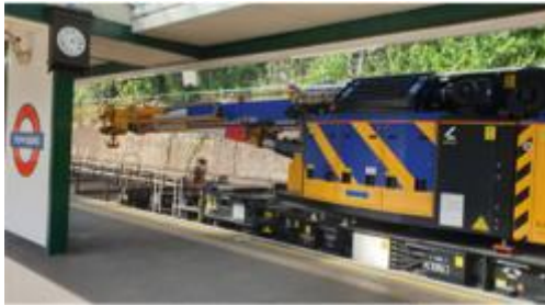
Figure 9: Kirow crane passing South Ealing station
