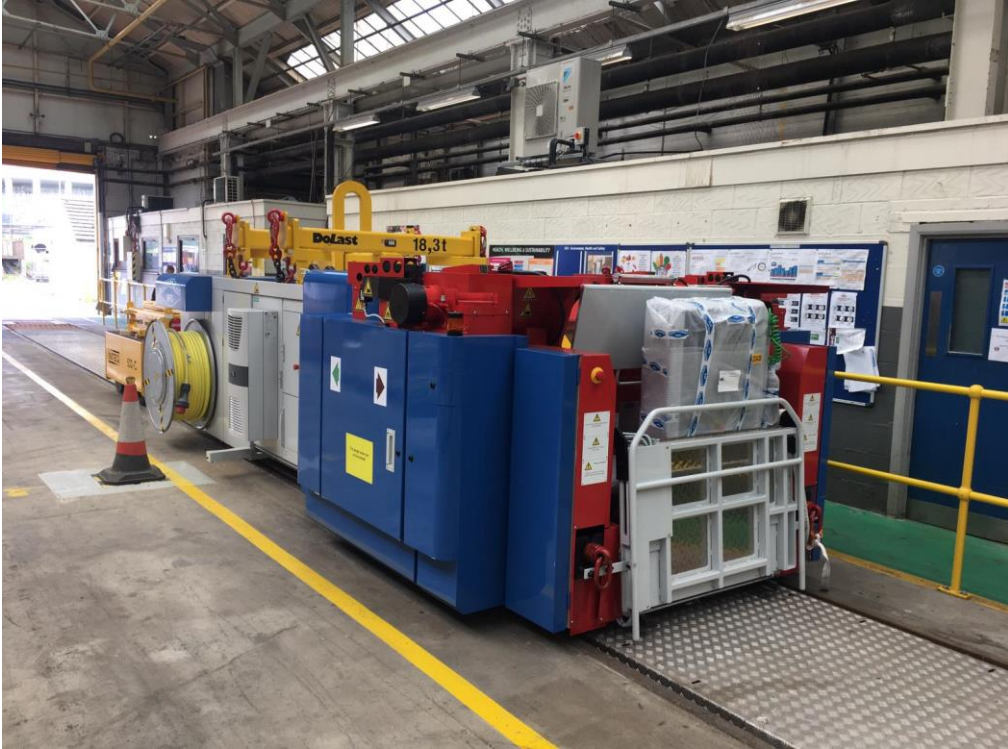
Images 4 and 5 - Mobile wheel lathe in use on 95 TS train at Morden depot Northern line
