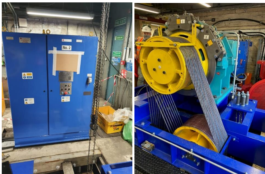
Figure 2: Installation of new lift ropes and controller at Belsize Park
