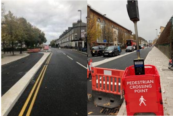
Image 1: C4 Evelyn Street construction
