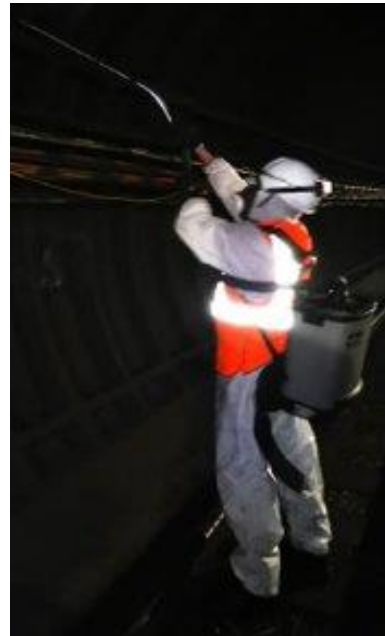
A colleague using a 'Bac-Vac' to clean a Tube tunnel
