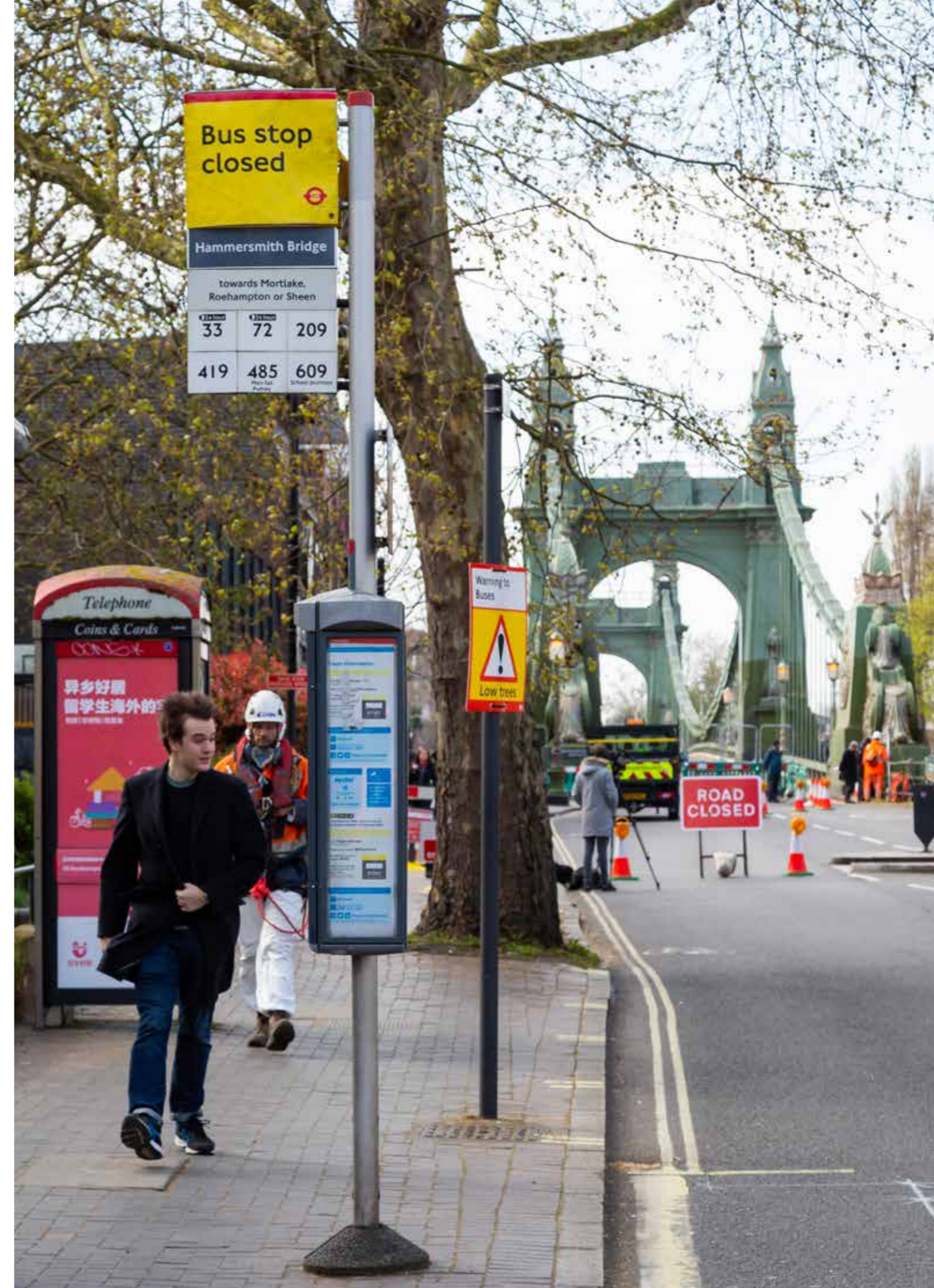
Hammersmith Bridge stabilisation work is under way
