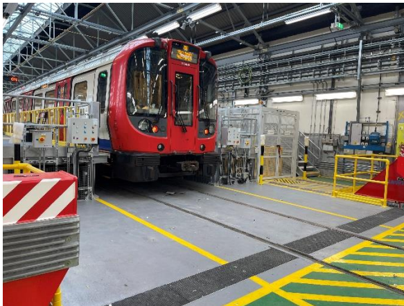
Figure 2 – S Stock train integration at the new Long Shed at Neasden Depot
