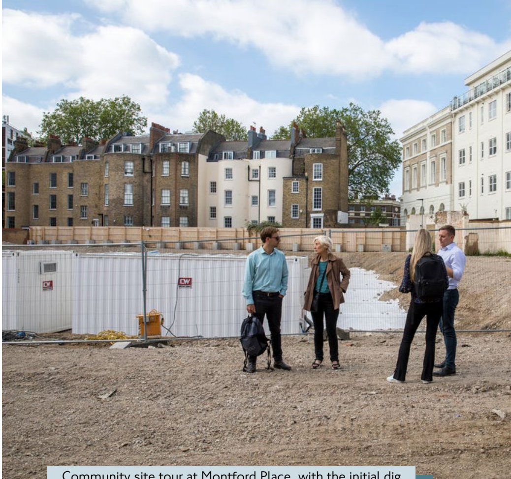
Community site tour at Montford Place, with the initial dig covered in plastic sheeting to prevent dust issues
