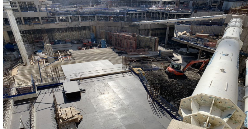
Construction site for the new station box at Elephant & Castle
