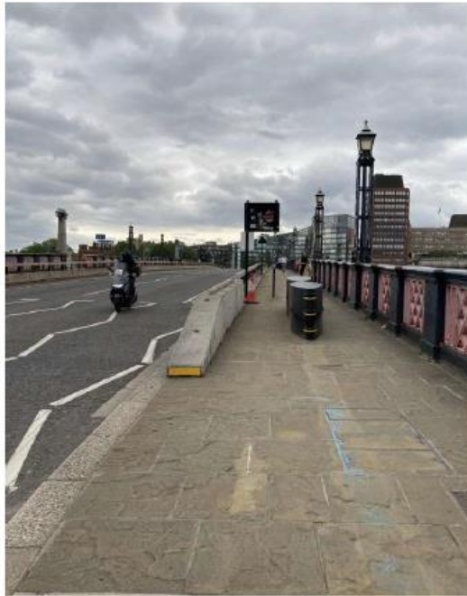
Figure 4: Temporary HVM along Lambeth Bridge
