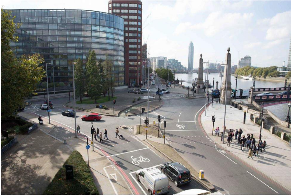
Figure 3: Existing layout of Lambeth Bridge southern junction, facing south towards Albert Embankment
