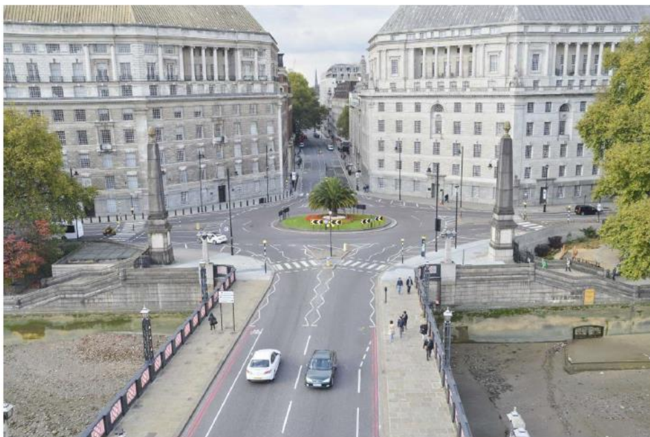
Figure 2: Existing layout of Lambeth Bridge northern junction, facing west towards Horseferry Road
