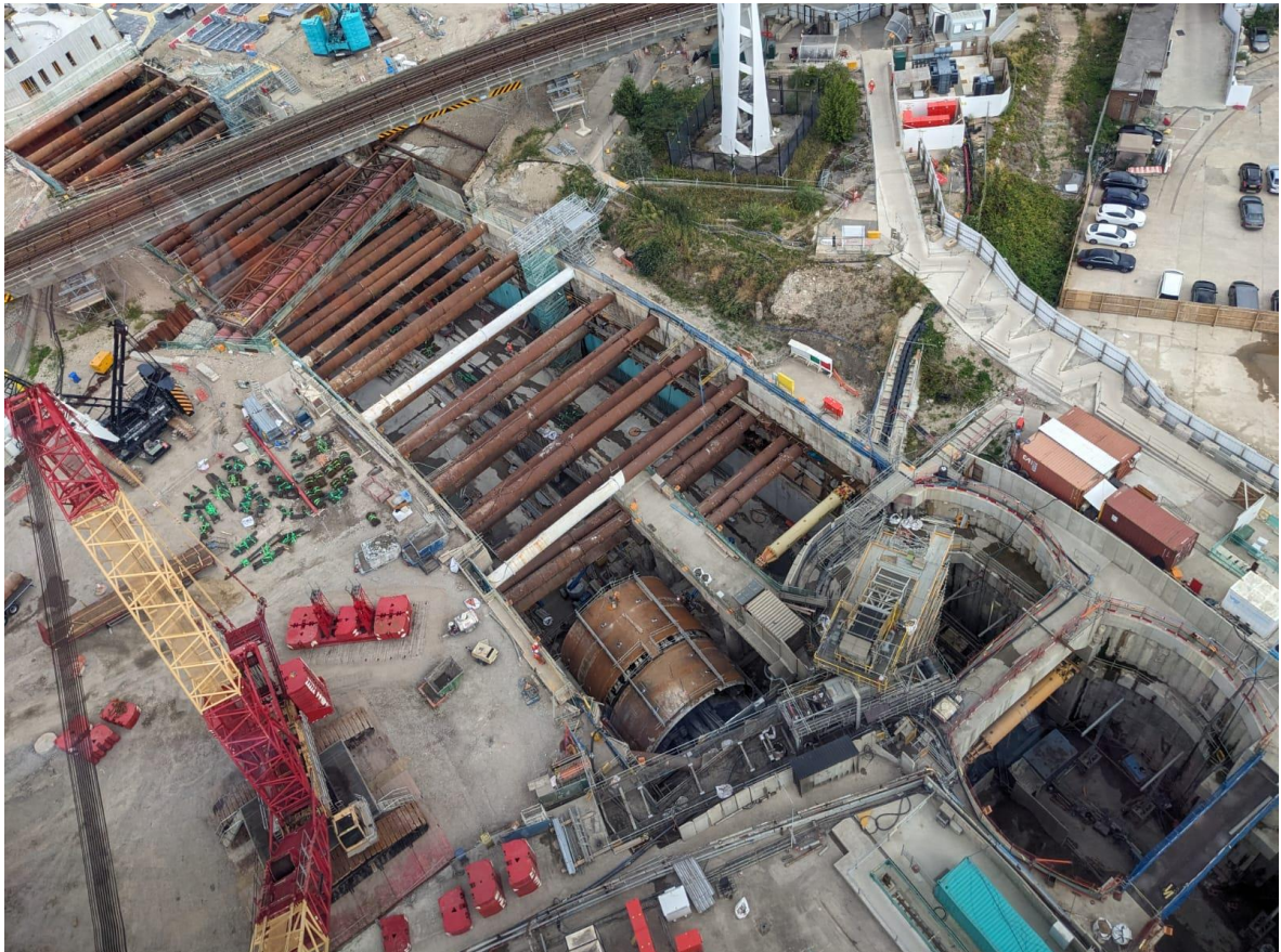
TBM “Jill” in the Newham retrieval chamber having completed all tunnelling
