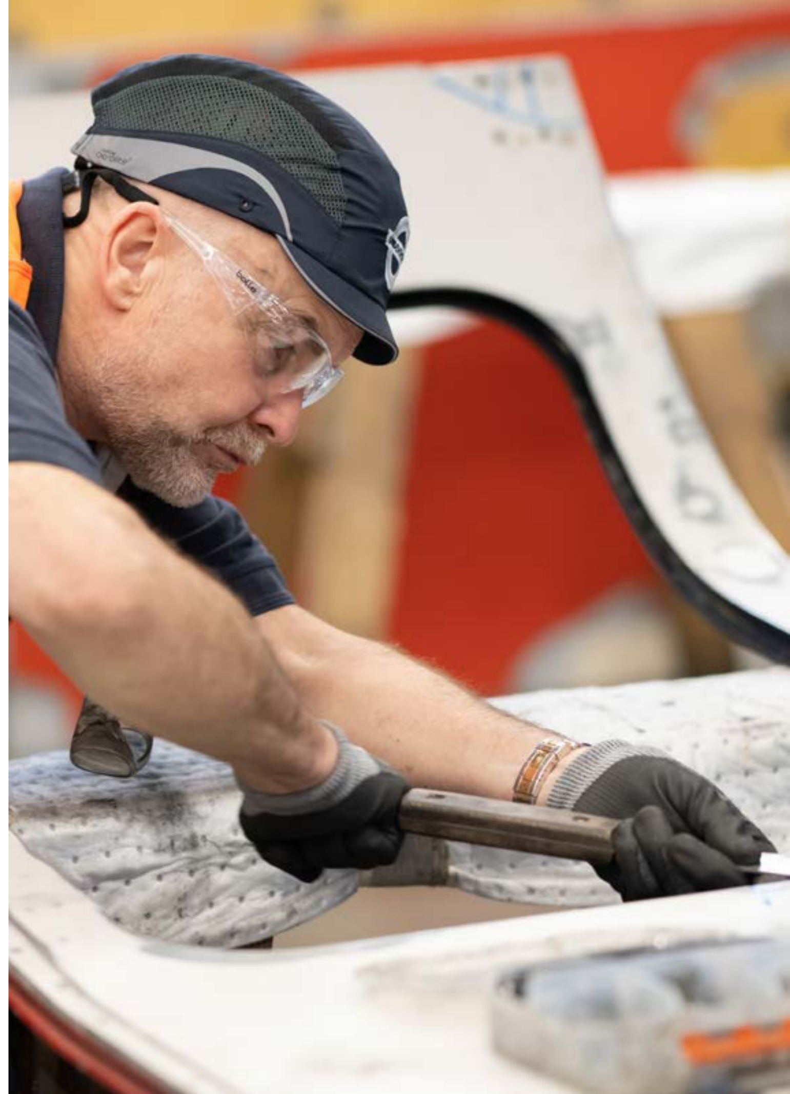
We've made strong progress on track renewals
