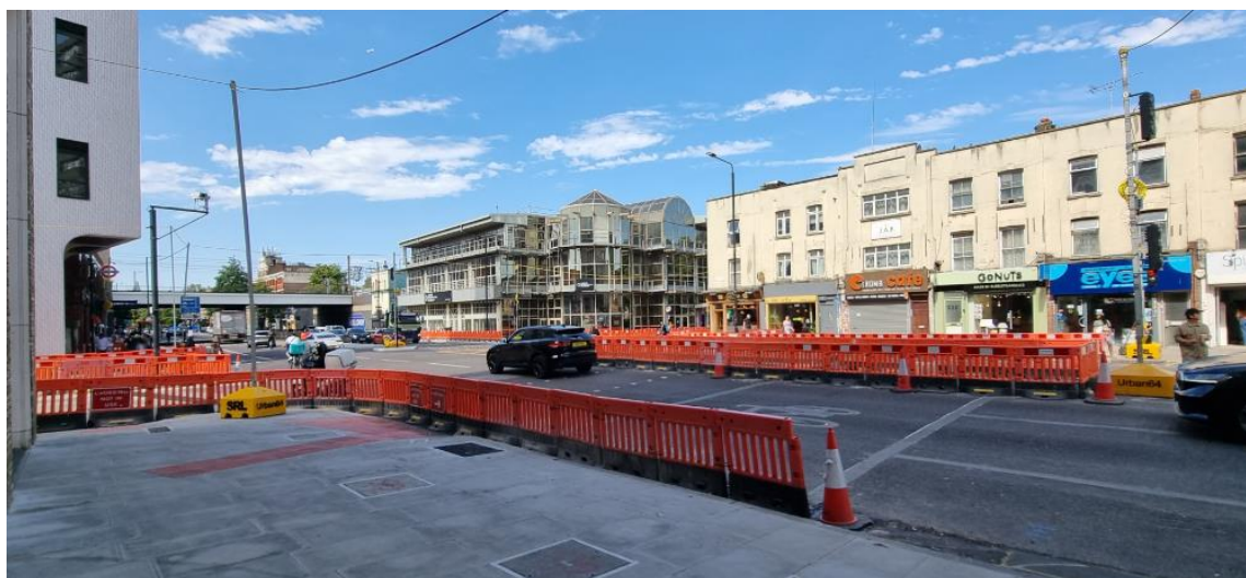
Figure 9 - Construction underway on Holloway Road Safer Junction
